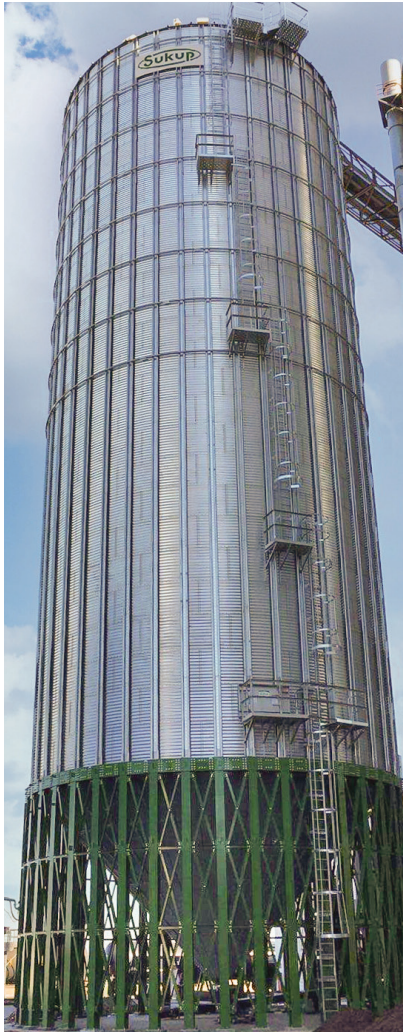
World's Largest Hopper Bin 42', 27- ring 128,000+ Bushel North Dakota October 2017
